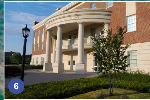
6 JERRY R. JUNKINS ELECTRICAL ENGINEERING BUILDING
