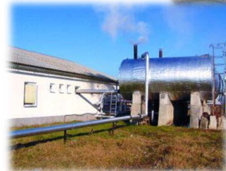
Degasification unit at Kunszentmárton, Hungary (Geothermal Era-Net)
