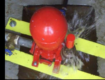
Water Ram Irrigation System
