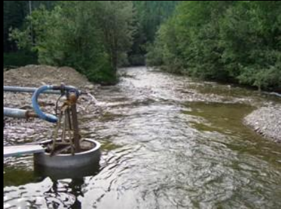
Monument Creek Provides Cooling Water (~40F)
