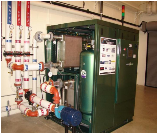
Industrial Boiler in Michigan
