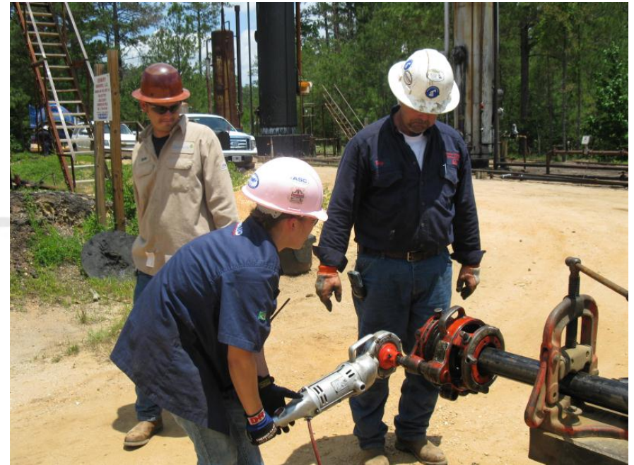
Knockout tank plumbing (supply) being installed
