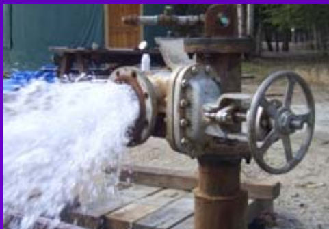
Geothermal Wells Provide Hot Water (~165F)
