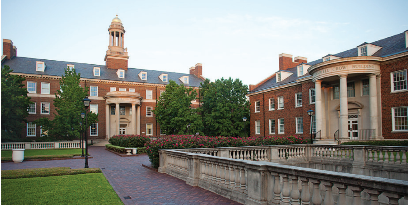
SMU Cox has announced plans to enlarge and modernize its three-building complex on Bishop Boulevard
