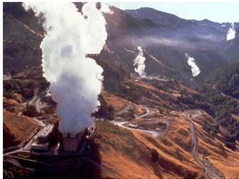
plants consist of excess steam and very small amounts of sulfur dioxide, hydrogen sulfide, and carbon dioxide. Because there is no combustion taking place, the levels of these gasses are much lower than emissions from fossil fuel fired power plants.
