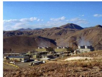
injected back into the Earth so that the process can be renewed over and over again. An example of an area using a flash steam operation is the CalEnergy Navy I flash geothermal power plant at the Coso geothermal field.
